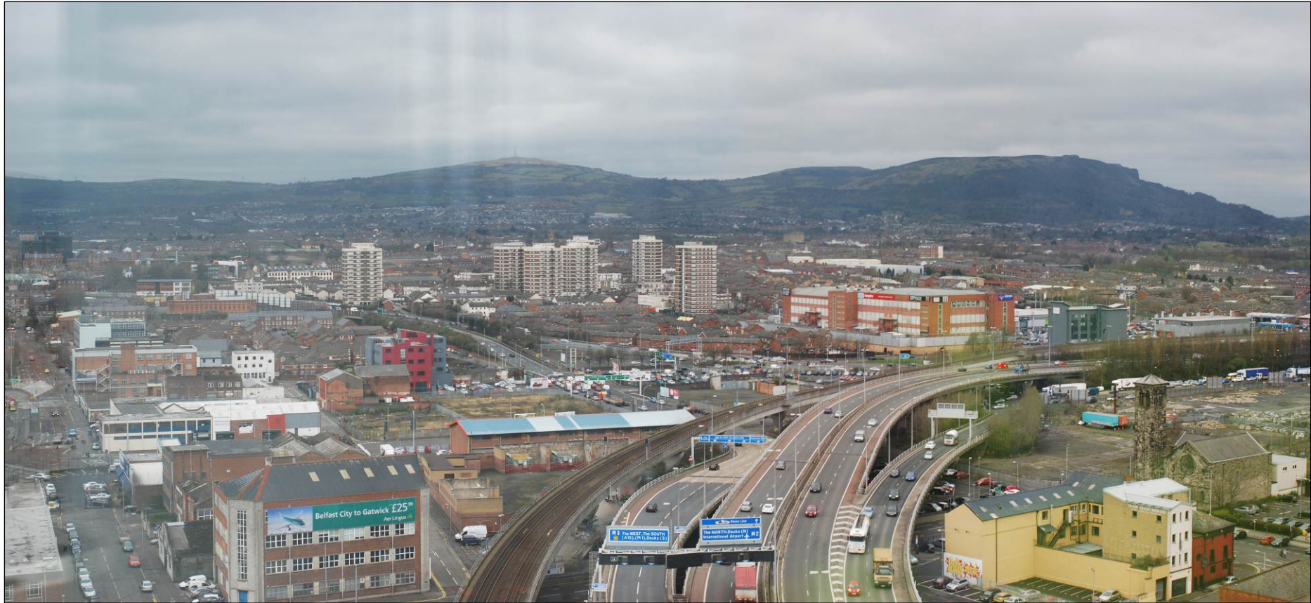
IMAGE 12 (Viewpoint 12): Existing view from Obel Tower of the existing road infrastructure.
